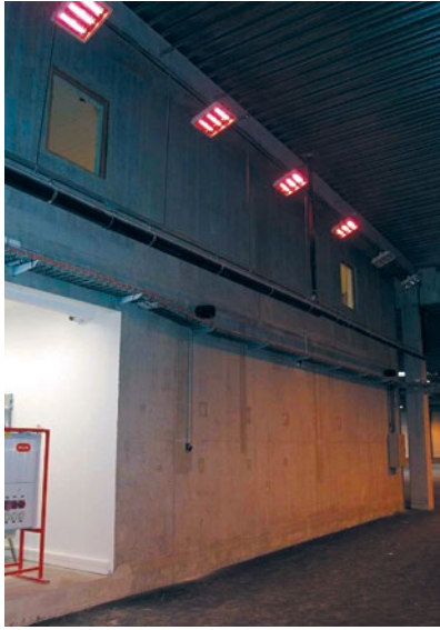
IRC can be mounted on the wall or on the ceiling and is suitable in buildings which are used sporadically like this go-cart track starting area.
