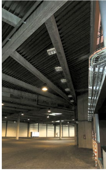
IRC can be mounted on the wall or on the ceiling and is suitable in buildings which are used sporadically like this go-cart track starting area.
