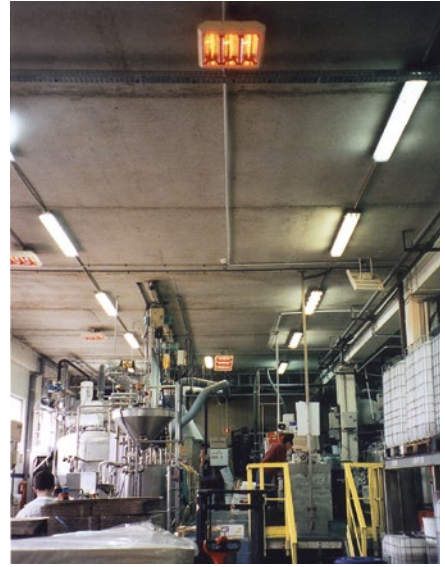
IRC is often installed in large warehouses. They give instant and effective heat which make them profitable quickly.
