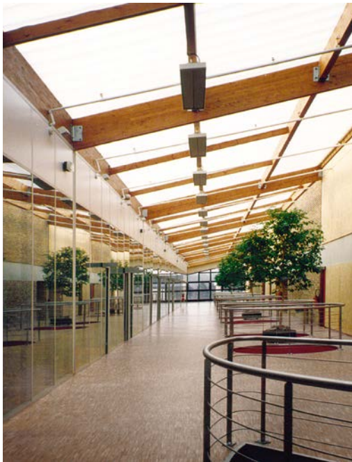
Corridors can be difficult to heat, but ceiling mounted EZ100 give off heat just where it is needed.
